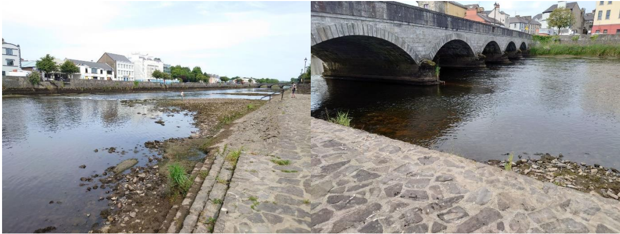
Site M5/6 Cathedral Pool - Existing bank defences and instream habitat with deflectors (low tide) (22 July 2021)
