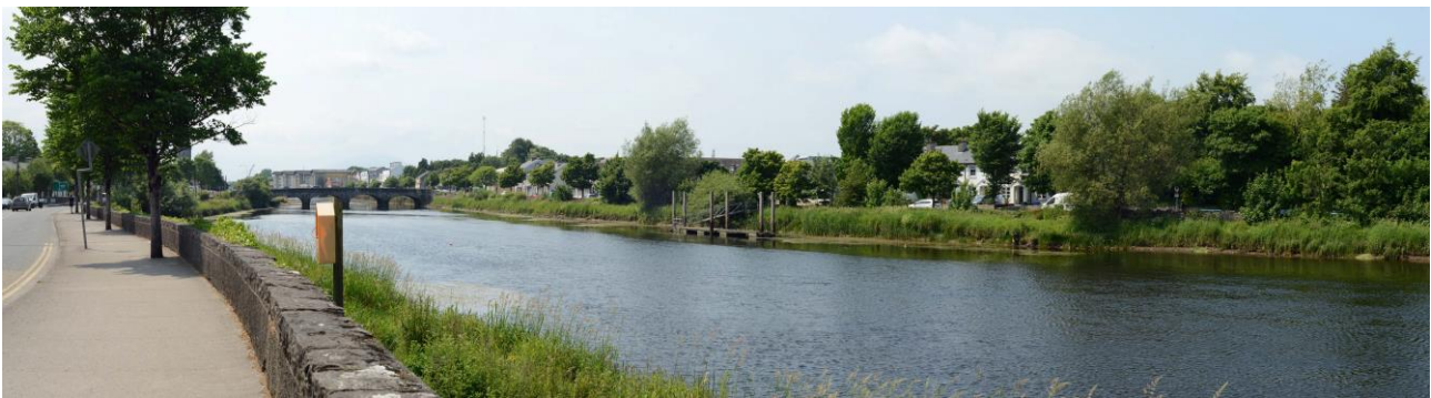
Figure 3-7 River Moy Existing Infrastructure – Looking U/S from Clare Street (RHS – Bachelors Walk/ LHS – Clare Street)
