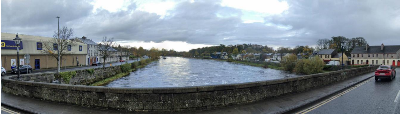
Figure 3-6 River Moy Existing Infrastructure – Looking D/S from the Lower Bridge (RHS – Clare Street/ LHS – Bachelors Walk)
