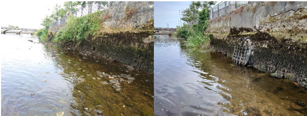
Site M9/10 Existing River walls on Ridgepool RHS and non-return culvert flap (22 July 2021)
