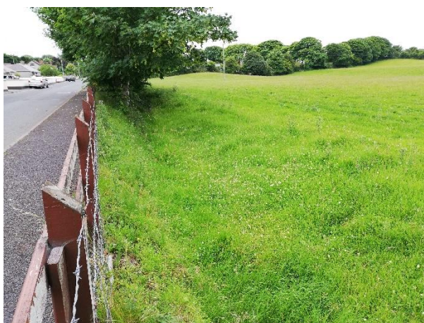
QG3 – Quignamanger, roadside stormwater swale (11 July 2022)
